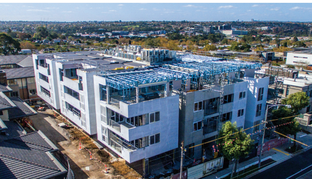
mecwacare's luxurious Robin Syme Residences in Malvern quickly took shape as we raced towards a spring completion date. A drone captured this photo of the retirement living complex, bathed in autumn sunshine. For more information, visit www.robinsymemalvern.com.au
