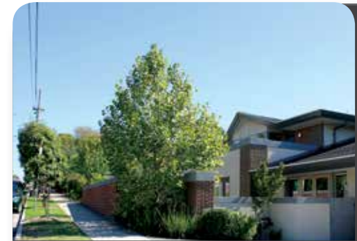
mecwacare Malvern Centre, Malvern Accommodates 100 residents
